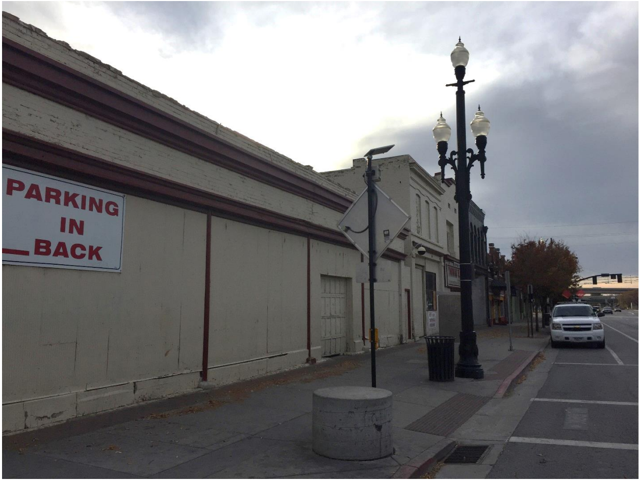
Photo 5: Looking west, along 200 South
